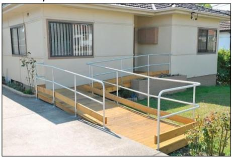
Figure 8: Ramp and handrails
