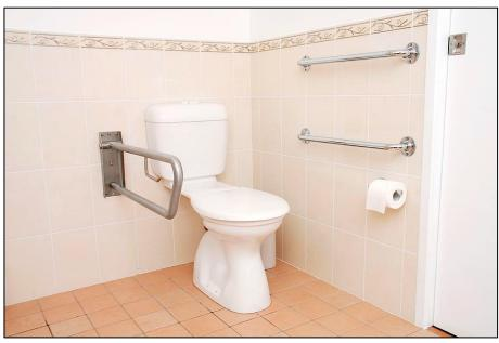
Figure 7: Grabrails in bathroom
