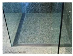
Figure 3. Grate drain in a shower recess (Stormtech, 2005)
