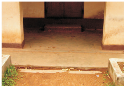
Fig 18 - Open drain blocks pathway and needs to be stepped across to reach destination
