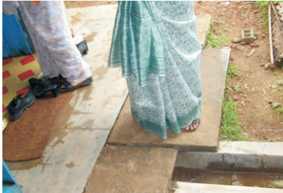
Fig 17 - Open drain too close to pathway
