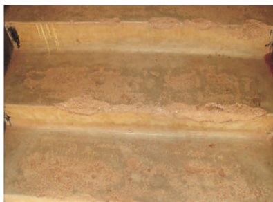
Fig 26: These steps are wearing away fast, creating a trip hazard.
