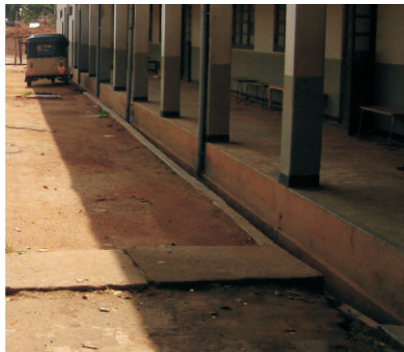
Fig 19 - Open drain directly below exposed edge of corridor
