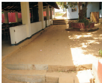
Fig 31: Steps along this path of travel make it inaccessible. The ground is relatively hard and tough..
