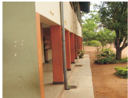
Fig 20 - Drainpipe opens to steps
