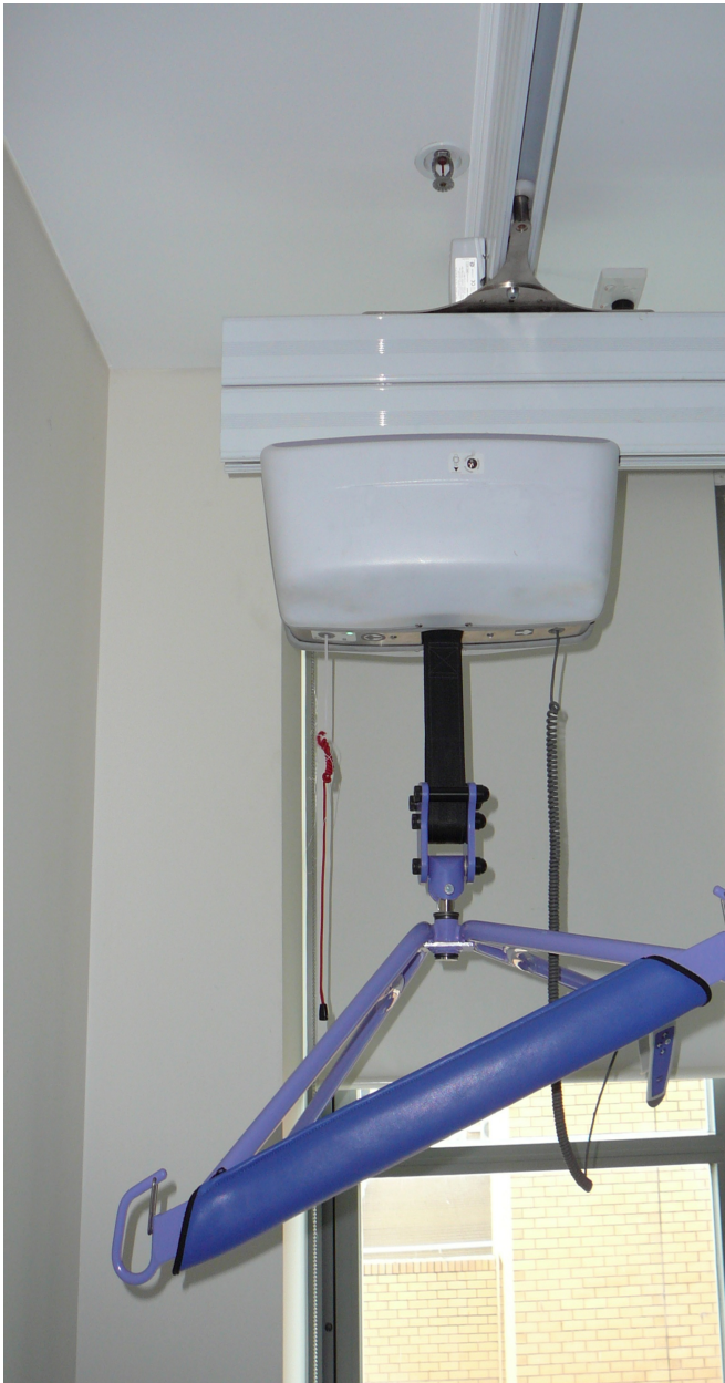
Figure 2: Example of a permanent hoist that does not use wands and hooks. There are also lifting modules with a quick-release system that allows the relocation of the lifting module to another location.
