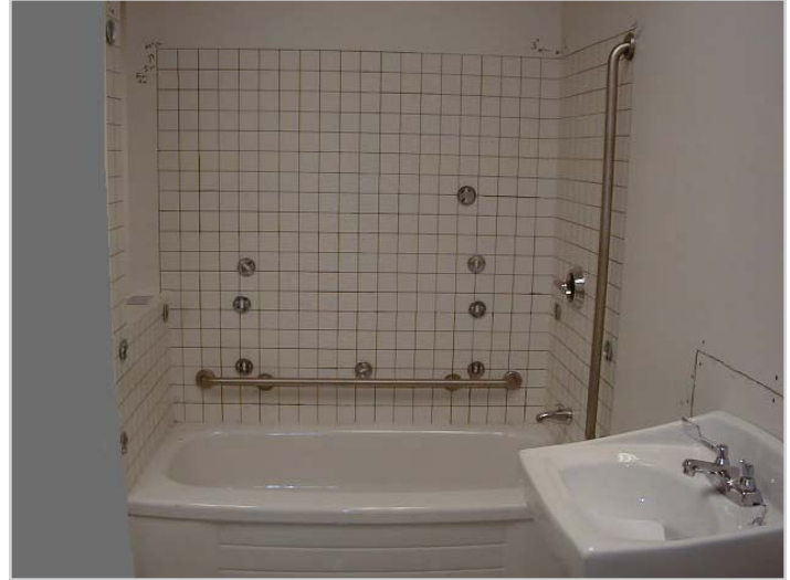
Figure 2 Grab bar configuration: Canadian Standards Association (CSA)
