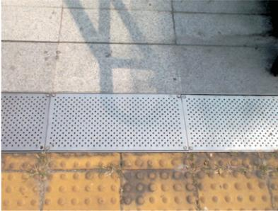
This drainage system is used in Thailand at the bottom of steps and ramps, and on the landings of ramps. It lies flat with the ground and the holes are not too big to catch mobility devices.
