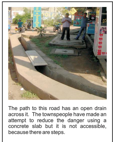
The path to this road has an open drain across it. The townspeople have made an attempt to reduce the danger using a concrete slab but it is not accessible, because there are steps.
