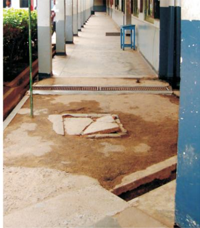
This pathway has a concrete bridge to cover a drain in the foreground—however it is only half covered! Next, there is a broken slab causing a trip hazard. Finally, there is grating with narrow gaps (good) to cover a drain. A mix of 'good' and 'poor' access
