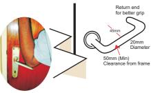
A lever door handle can be opened with an elbow if the fingers and hand cannot grasp.
