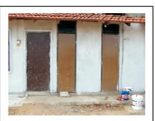
Three doors are shown. None are wide enough for wheelchair access. There are no proper handles that are easy to grasp. The pathway in front of the doors is too narrow to allow easy turning into the doors. There is also a step up to each of the doors.
