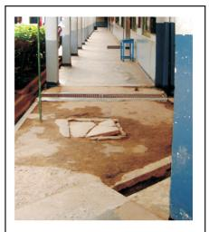
This pathway has a concrete bridge to cover a drain in the foreground—however it is only half covered! Next, there is a broken slab causing a trip hazard. Finally, there is grating with narrow gaps (good) to cover a drain. A mix of 'good' and 'poor' access
