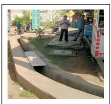
The path to this road has an open drain across it. The townspeople have made an attempt to reduce the danger using a concrete slab but it is not accessible, because there are steps.
