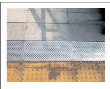
This drainage system is used in Thailand at the bottom of steps and ramps, and on the landings of ramps. It lies flat with the ground and the wholes are not too big to catch mobility devices.
