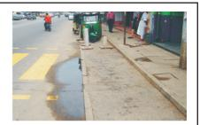
**PROBLEM: NO CURB RAMP** Curb ramps should be at either side of a pedestrian crossing.
