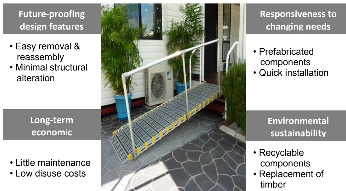
Figure 3. Qualities of demountable ramp for flexible home modification
