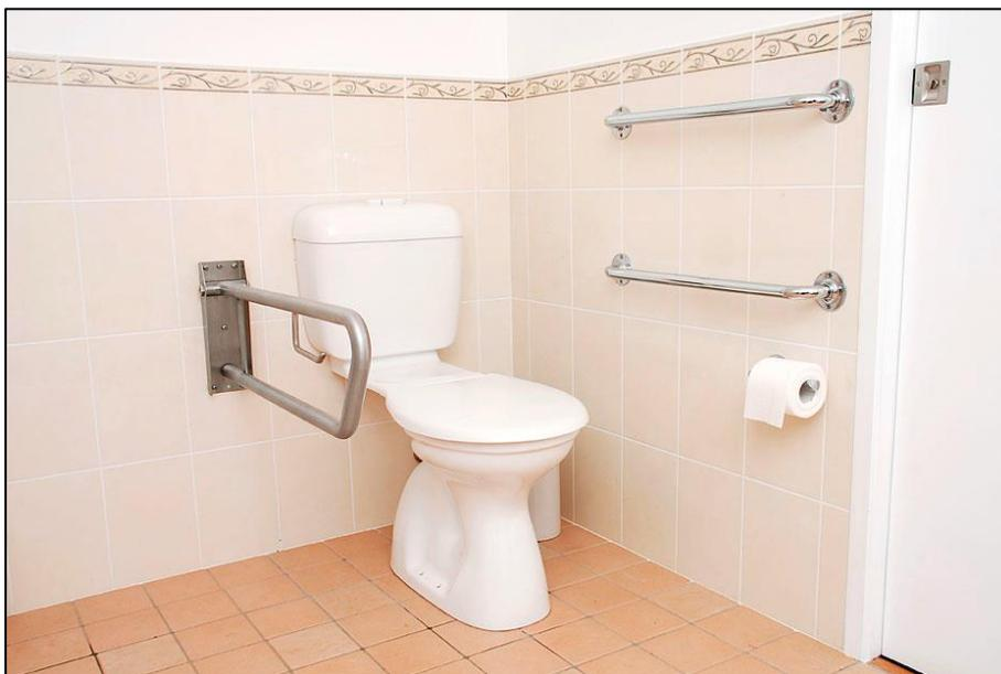
Figure 7: Grabrails in bathroom
