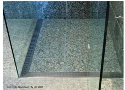
**Figure 3. Grate drain in a shower recess (Stormtech, 2005)**
